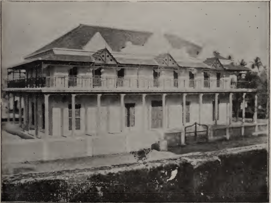
NEW HOSPITAL, MADURA.
